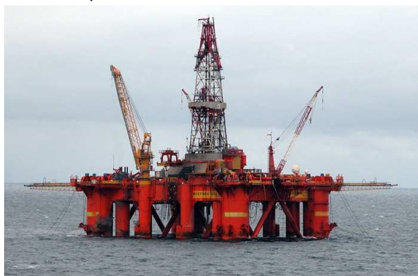
Fig. 3 LNI Swissgas generators are installed on the most critical locations
